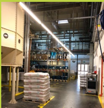
Coffee roasting plant “before” with old lighting
